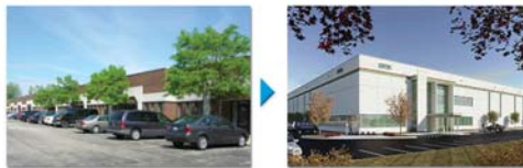
From Incubator Office to New 100,000sf Build-to-Suit Sales & Distribution HDQs
